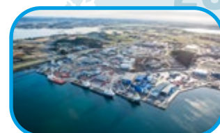
Next generation supply base in Tananger.
